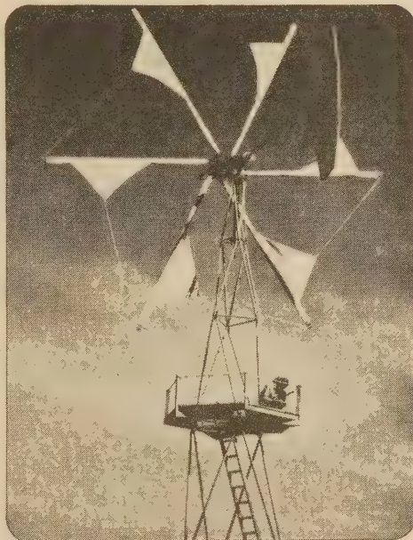
BOTH THESE WINDMILLS USE OCTAHEDRON TOWERS
